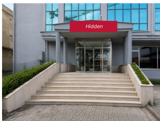
Stairs to main building entrance
